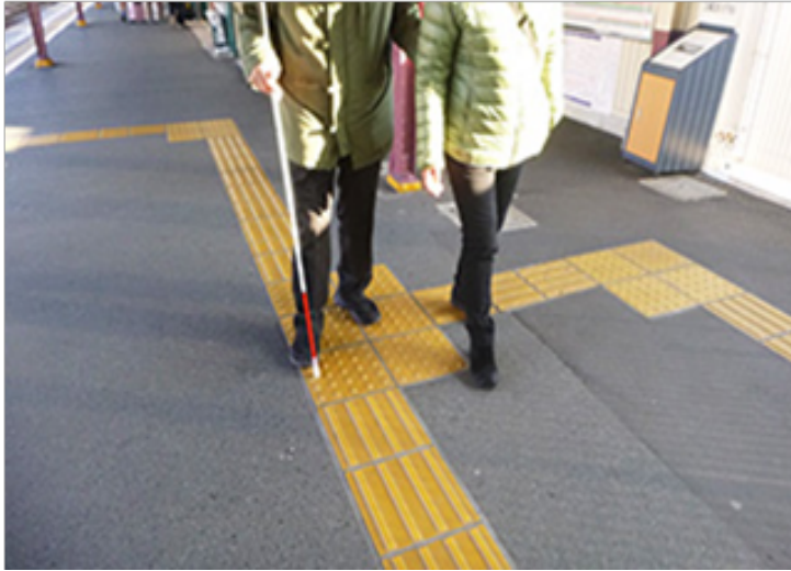
Fig. 5. Indoor braille block use for accessibility information of Japan
