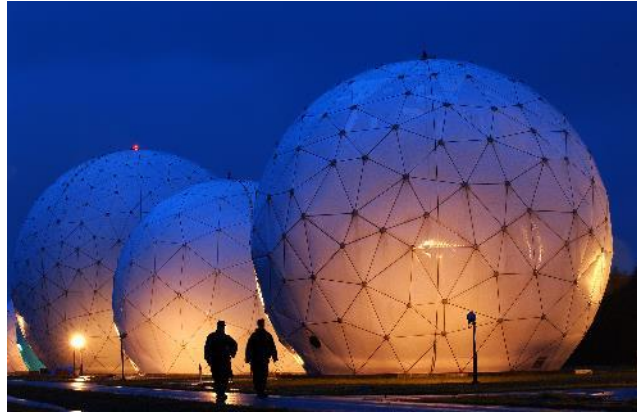
Spherical Radar Radome
