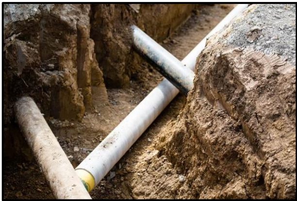
Figure 1: Pictures showing current status; manual excavation near existing pipes and protection with wood pieces
