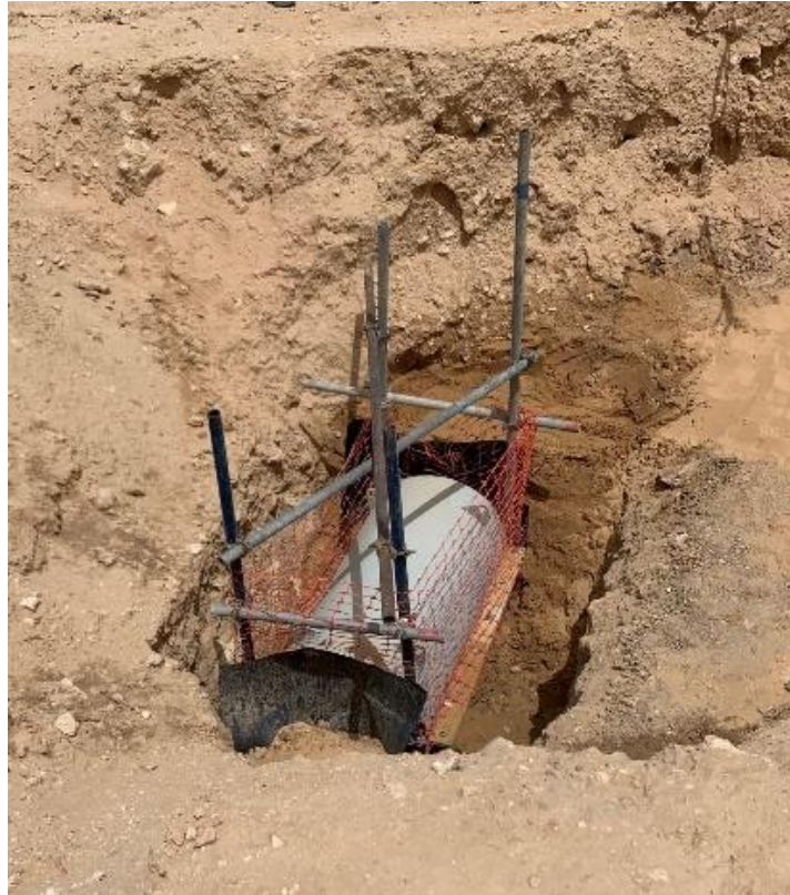
Figure 6: Protection tool assembled in place around the pipeline at the crossing location
