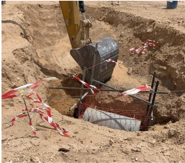
Figure 7: An excavator was used to remove sand and soft soil around the pipe to dig a crossing trench
