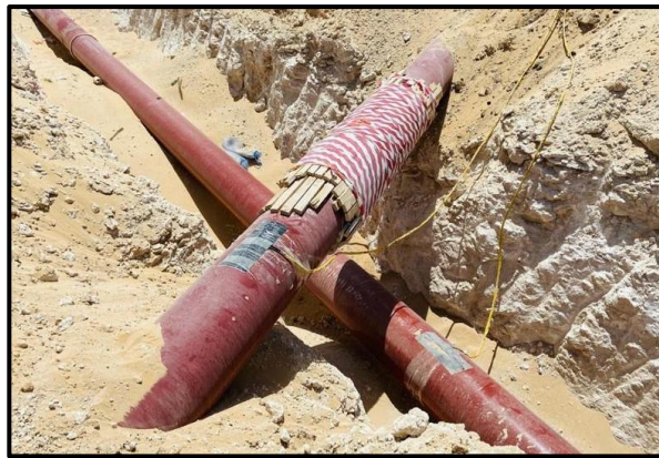
Figure 1: Pictures showing current status; manual excavation near existing pipes and protection with wood pieces
