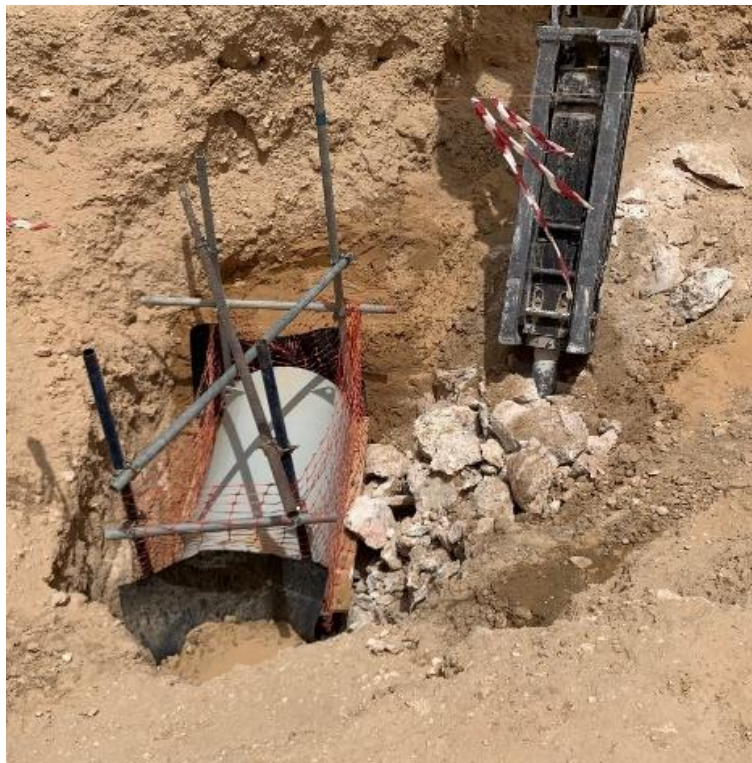
Figure 8: A rock breaker was used to dig a crossing trench for the new pipeline
