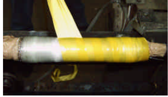
Fig. 9: Wrapping with fabric tape
