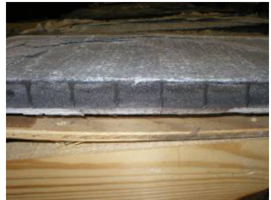
Figure 6: 7.5CM CARBON FOAM PANEL INTACT AFTER FIRE
