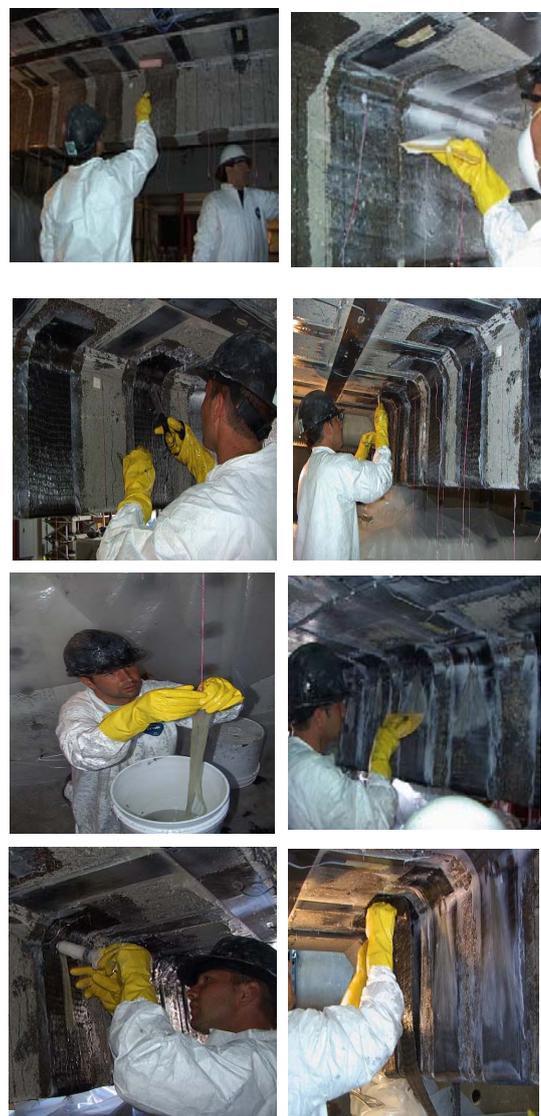
Fig 9: Placement of FRP stirrups and anchors
