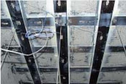
Fig. 6(a): Section of deck rehabilitated with prefabricated strips
