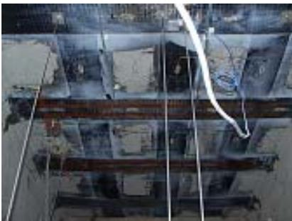
Fig. 6(b): Section of deck rehabilitated with wet layup of unidirectional fabric
