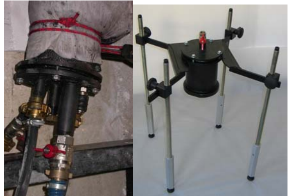
Fig. 11 Top and bottom pieces of the FuranFlex®
