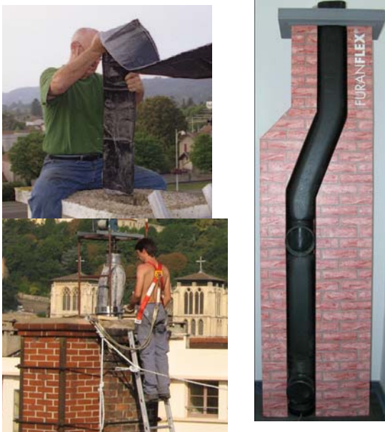
a) b) Fig. 7 Installation of the FuranFlex® tube (a); The hardened chimney (b)
