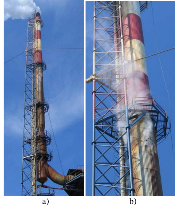
Fig. 15 Steel chimney (a), Steam escape (b)
