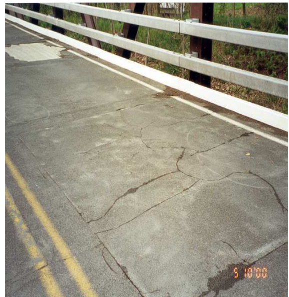
Fig. 1. Deteriorated a wearing surface material on FRP bridge deck [1]
