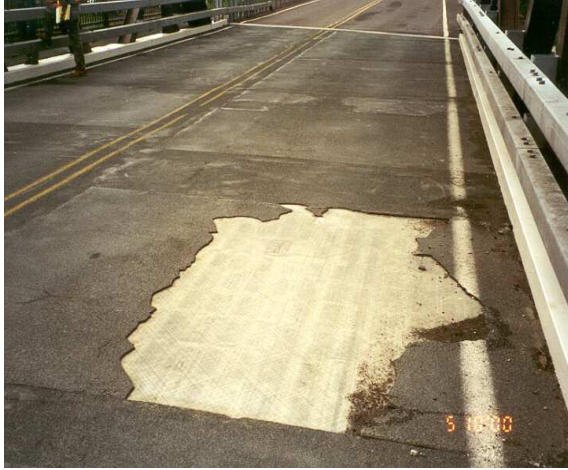
Fig. 2. Delamination of a wearing surface material on FRP bridge deck [1]
